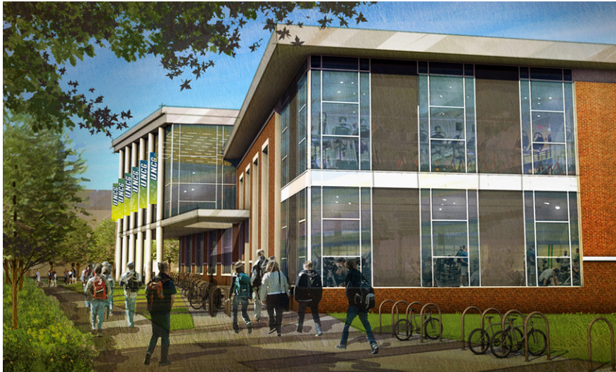
Leonard J. Kaplan Center for Wellness designed by RDG Planning and Design, under construction
